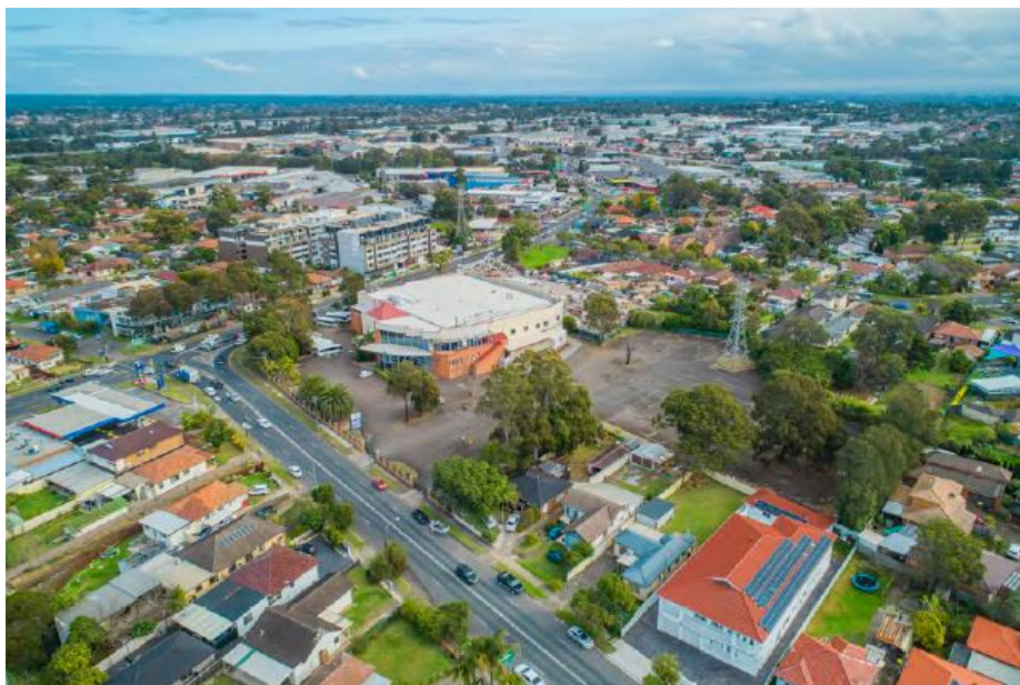
Figure 2. Current view to site looking southwest
